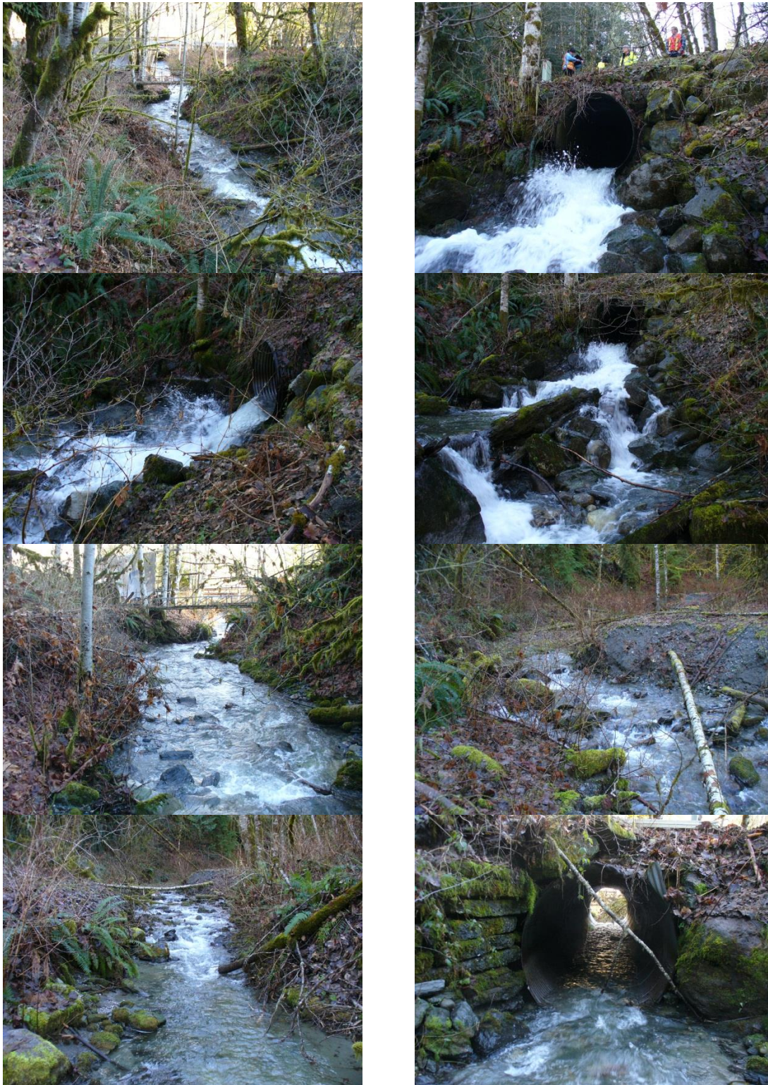
Figure 8 Christian Camp Road Culvert
