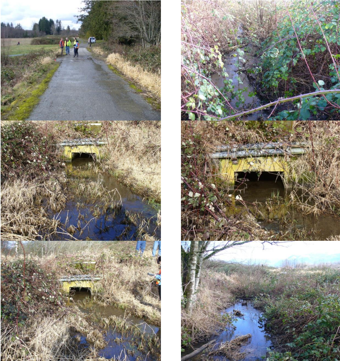
Figure 10. Dairy Tributary Culvert
