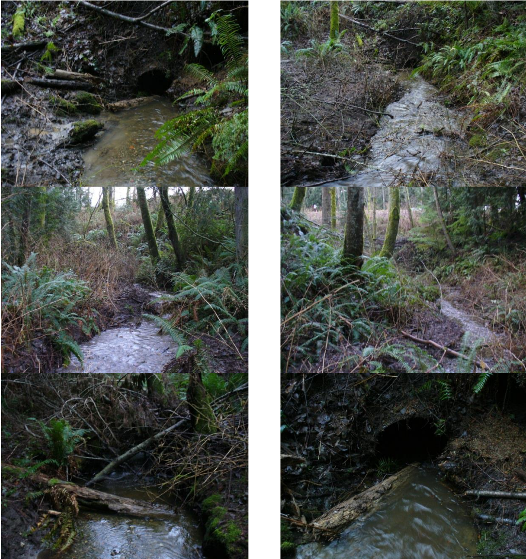
Figure 7: English Road Culvert
